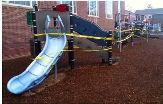
Playgrounds in need of repairs
